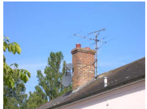
Below: unattractive aerials and satellite dishes
